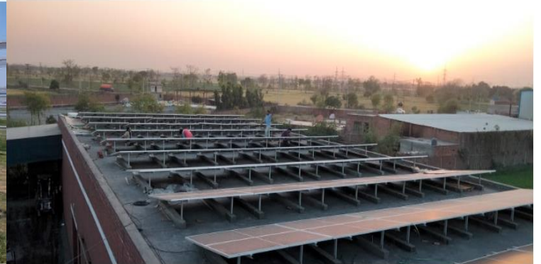
Flat RCC Roof (Non Elevated)
