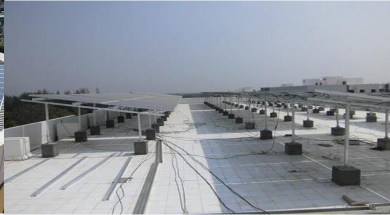
Flat RCC Roof (Elevated)
